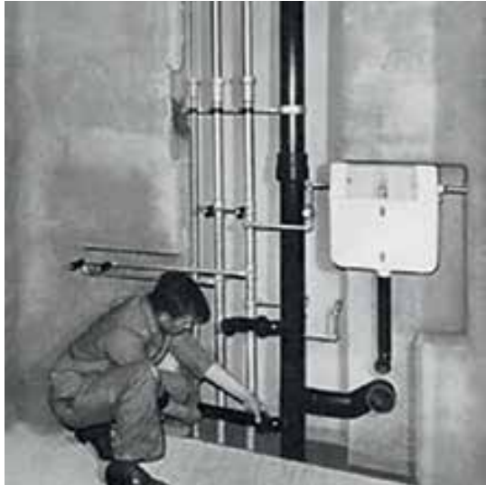
↑ Introducing the first concealed cistern in 1964
